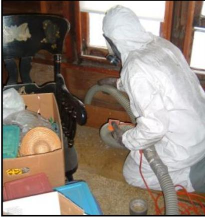
Cellulose insulation is installed in the attic and sidewalls of a home. Insulating a home is one of the most cost-effective energy saving measures.
